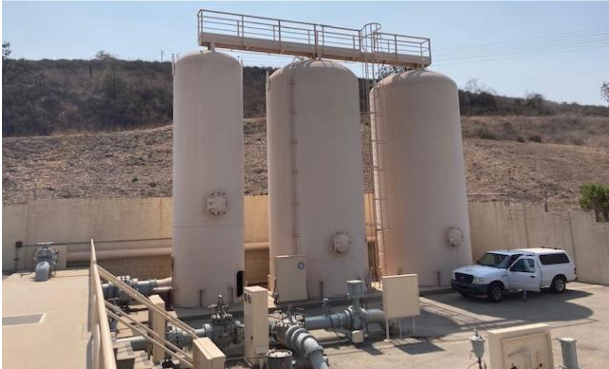
Figure 3 View of Surge Tanks, View Southeast
