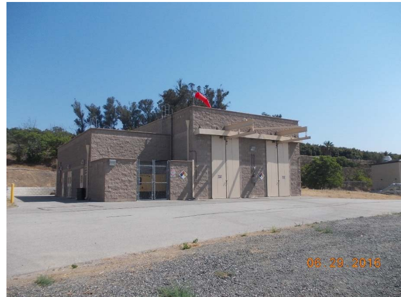
d. Wellfield disinfection building, example of masonry to be used
