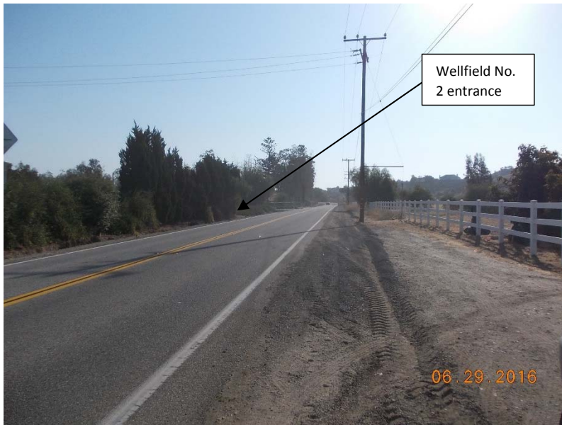
a. View from Grimes Canyon Road, with Wellfield no. 2 entrance
